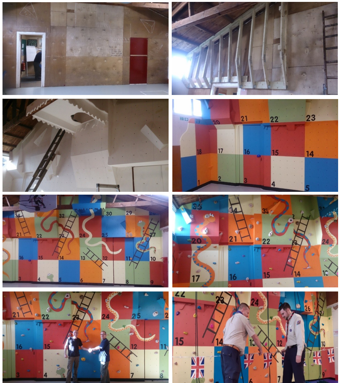
Left to right from top: The old wall; Framework; Primer and undercoat; Square grid and numbers; Snakes and ladders; Hand holds and belay points; Finished!; Opening ceremony
